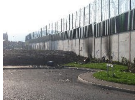
Previous damage to the wall during riots in recent years
